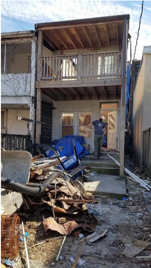
Image 8: 1426 Hollins Street – Rear of house, March 12, 2021
